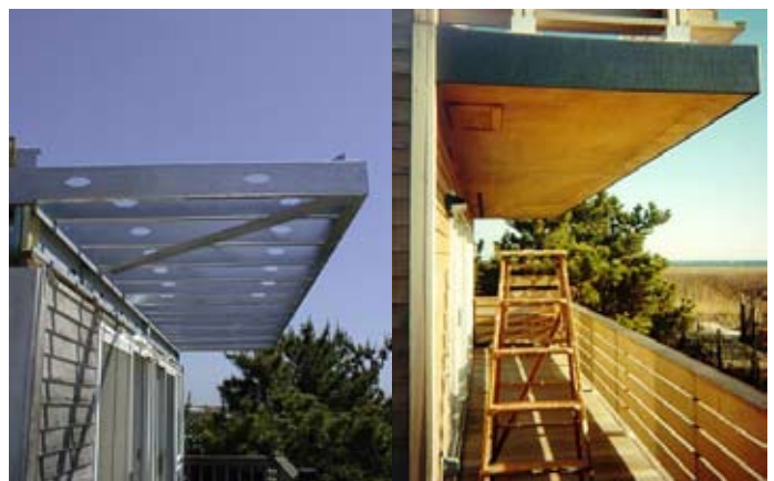
Figure 9 - New Jersey Site Under Construction
