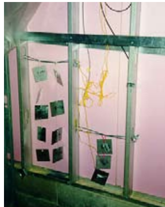
Figure 7 - Wall Cavity Specimens and Sensors in Hamilton, Ontario, Site
