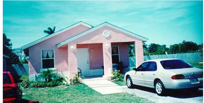
Figure 2 - Miami, Florida Corrosion Site
